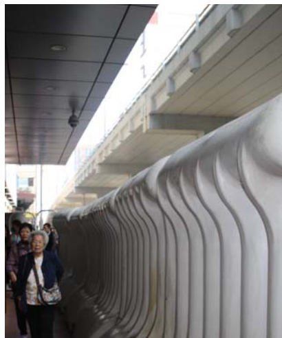
These are not decorative shapes. They're concrete barriers, ready to be moved into place to protect the police station if needed.
